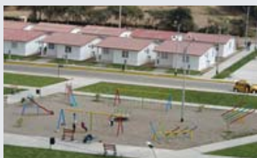
GHS housing solutions, like here in Chincha – Peru, offer affordable accommodations for a better life all around the world.
